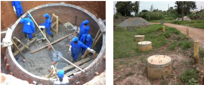
Figure 3: Construction of dome Shaped Digesters Source: Chris, 2008
